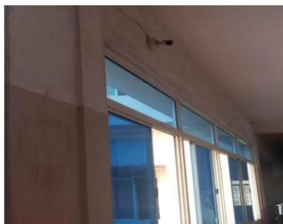
CCTV in Corridors
